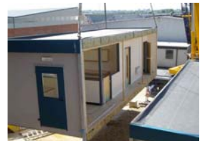
Lifting Into Position
